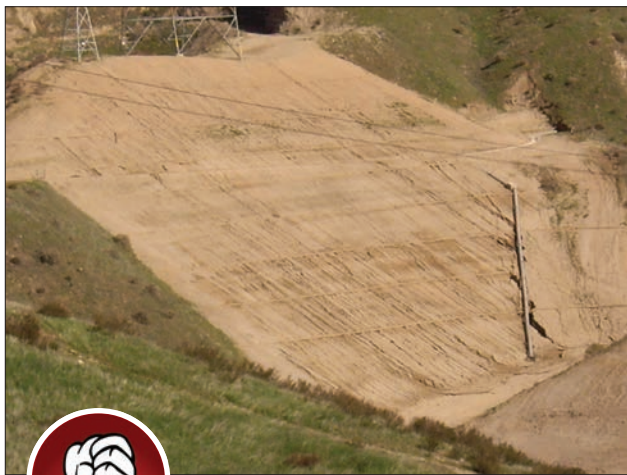
Fig. 2-3. This slope is exhibiting signs of rill erosion and additional BMPs are needed.
