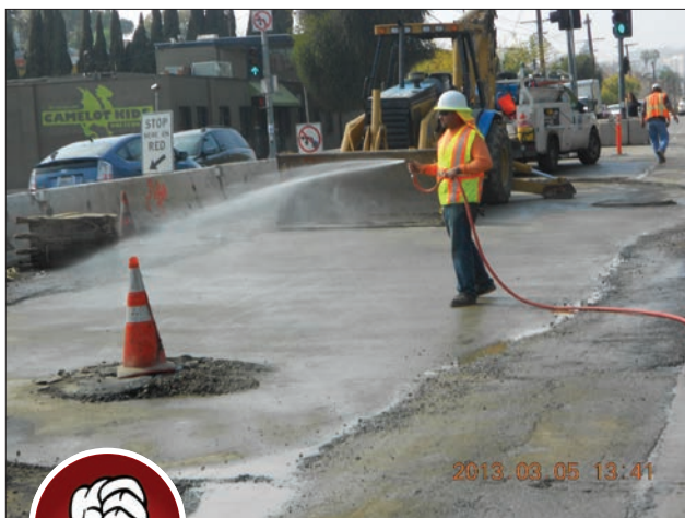
Fig. 2-11. Washing down the street after paving and concrete maintenance can create a non-storm-water discharge. Hand or mechanical sweeping is a better option. Source: RBF Consulting
