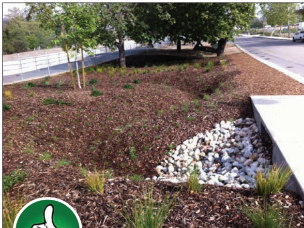
Fig. 2-8. No visible signs of erosion within the mulch areas or clogging indicate that this storm drain outlet is functioning well. Maintenance is not currently needed.
