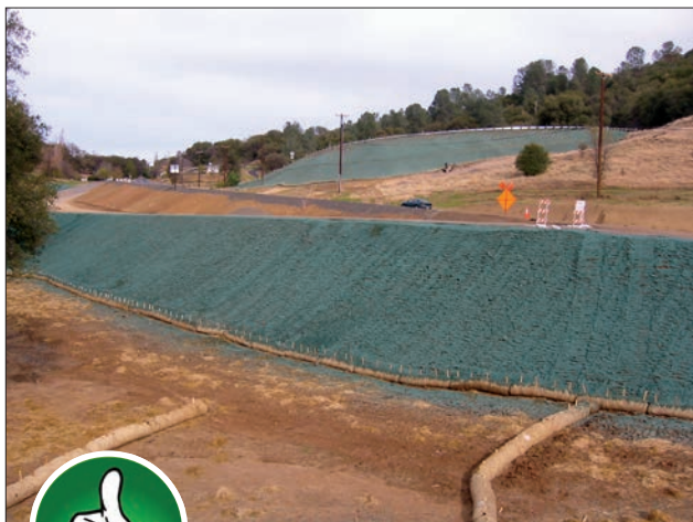
Fig. 2-6. No signs of surface depressions or erosion indicate that the binder used here has been adequately applied.
