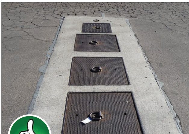
Fig. 3-12. Clarifiers such as this one are commonly utilized within wash rack areas.
