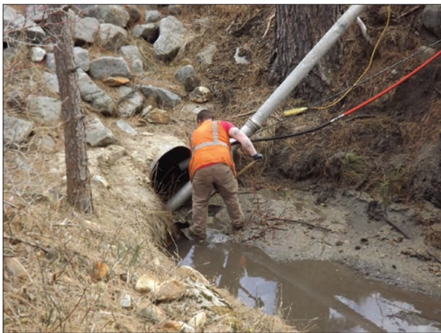
Fig. 2-1. Crews clean a culvert.
